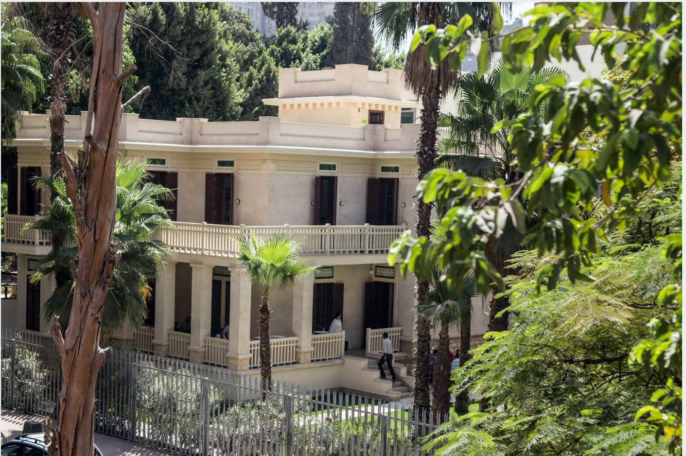
Building that was torn down and reconstructed, Roger Anis
